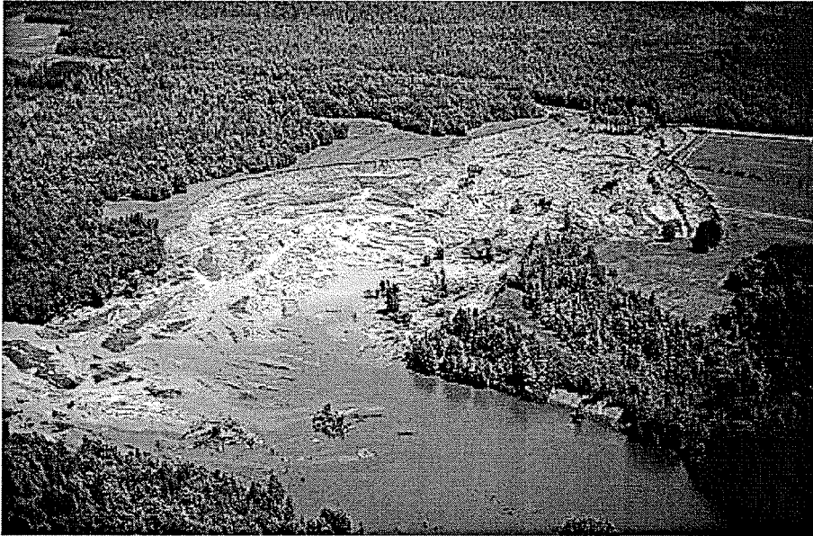
Figure 8. The Lemieux landslide several days after failure. Note the large intact rafted sections, and the severing of Regional Road 16. Some of the rafted blocks show rotation while the bedding in other blocks remains horizontal suggestive of lateral translation. The blocked South Nation River, flowing from right to left, is at the bottom of the picture. Photograph from the Geological Survey of Canada.
