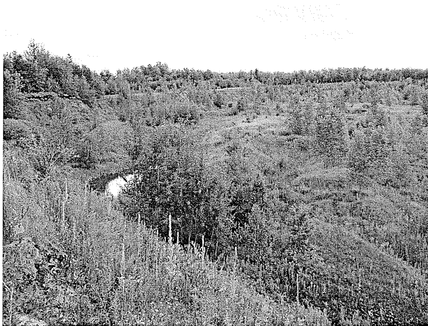
Figure 11. The Lemieux landslide crater in 2004, 11 years after the failure. Total crater depth is approximately 10-12 m. Notice the muting of the previously sharp-edged blocks of cap material. Revegetation of the crater is also well underway.
