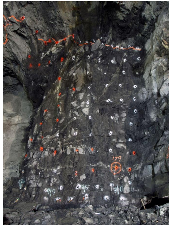
Figure 13 - Isoclinal recumbent folds of early SE-dipping foliation in Hartland formation (OCh) outlined by granitoid sills (g) with gently inclined penetrative foliation. Recrystallization during folding and shearing produces penetrative mica foliation (Feature 10.) that has formed parallel to compositional layering. Gently inclined foliation joints are prominent discontinuities ( J_1 ) and have formed parallel to the foliation and parallel compositional layering. These are intersected by steep NE-trending ( J_2 ) and NW-trending ( J_3 ) joints and faults producing overbreak seen at top of image. (Digital image taken 19 December 2012.)
