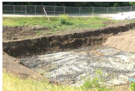
Figure 17. Another view of the clay layer showing the soil above it.
