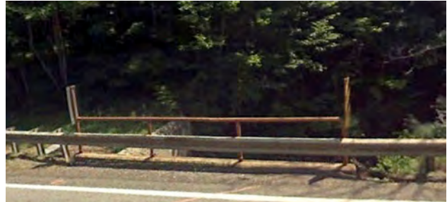
Figure 19. Bridge in 2009, before being rebuilt.
