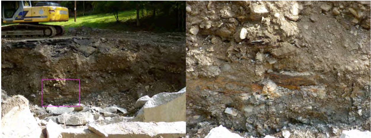
Figure 20. Subsurface beneath road a bridge under reconstruction. Area in highlighted rectangle is enlarged to the right.
